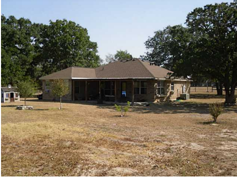
Back view of home
