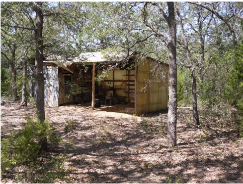
View of Shed
