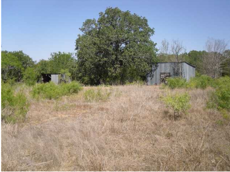
View of shed
